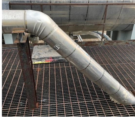
**Figure 17.** 45 degree 1.5D bend at launch
