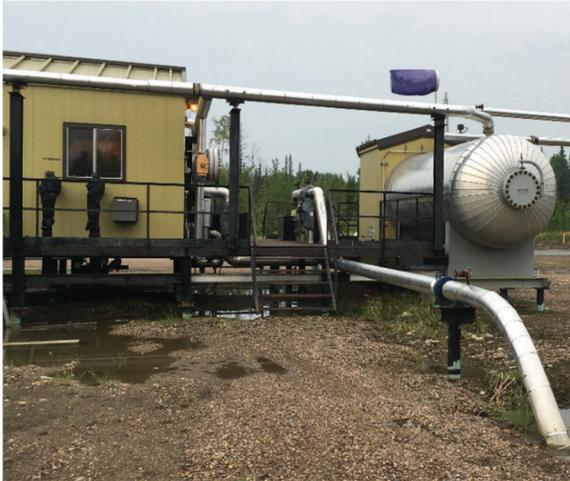
**Figure 16.** Overview of the launch site, 2 tight bends and sweep into the ground
