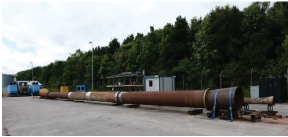
Figure 7: Pull rig in unloaded and supported condition.
