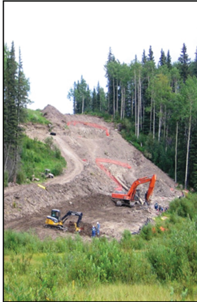
Figure 1: Landslide movement parallel to pipeline
