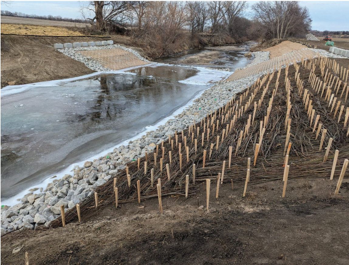
Figure 10. Partial Installation of The Brush Mattress and Live Stakes
