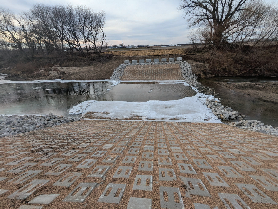
Figure 7. ACM System Spanning the ROW to Top of Banks
