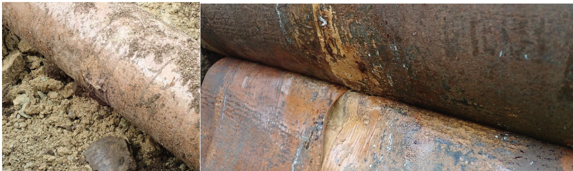
Figure 10: General Excavation Findings at Location 1
