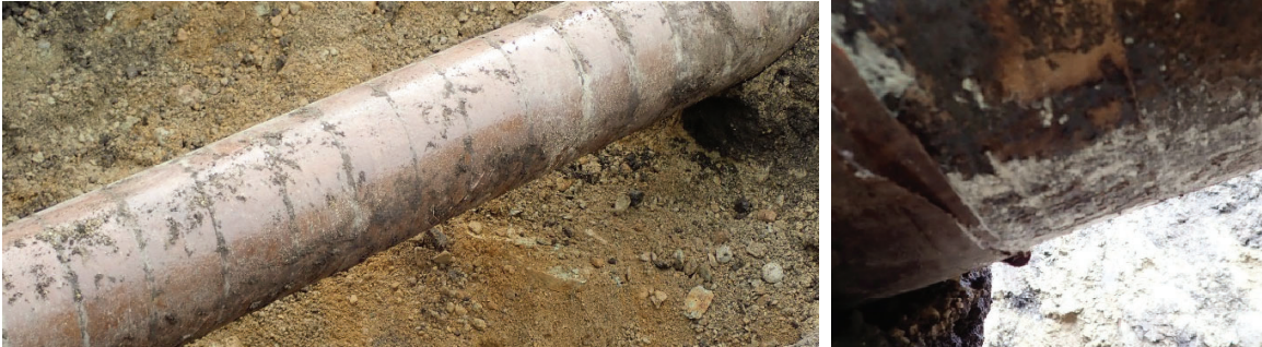
Figure 11: General Excavation Findings at Location 2
