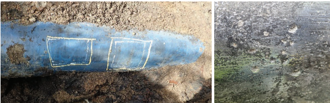
Figure 12: General Excavation Findings at Location 3
