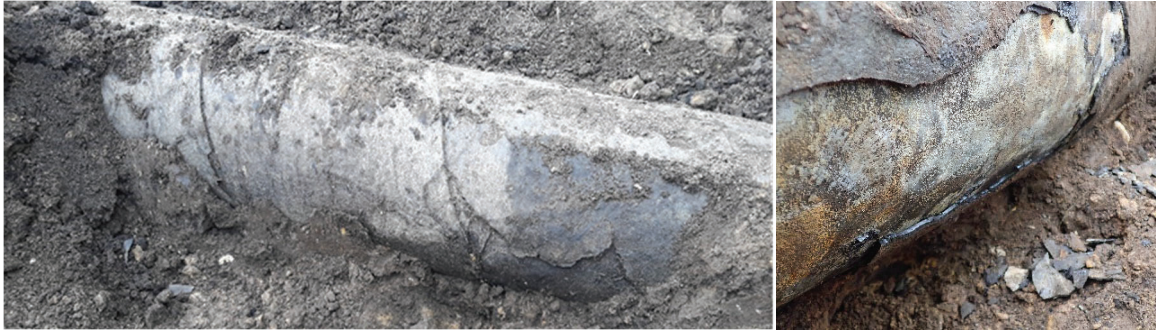
Figure 13: General Excavation Findings at Location 4
