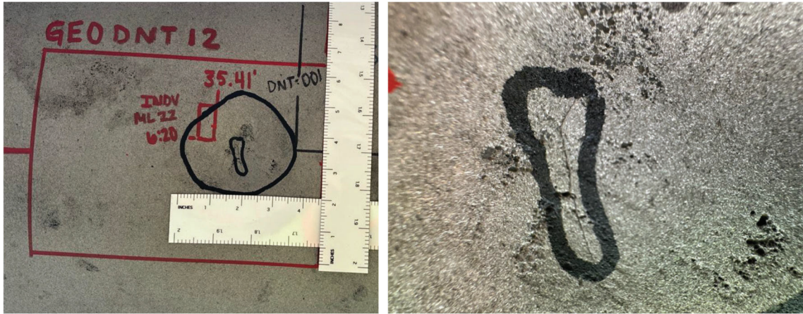
Dent with Metal Loss and Crack
