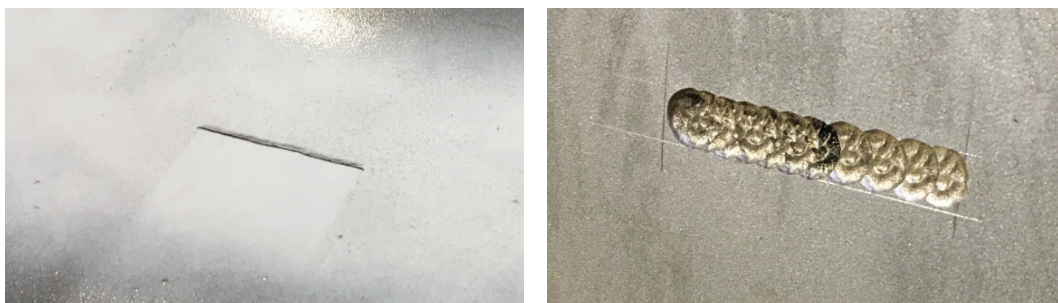
Figure 9. Example of a synthetic crack (made visible by MPI) and a synthetic sharp-edged corrosion.
