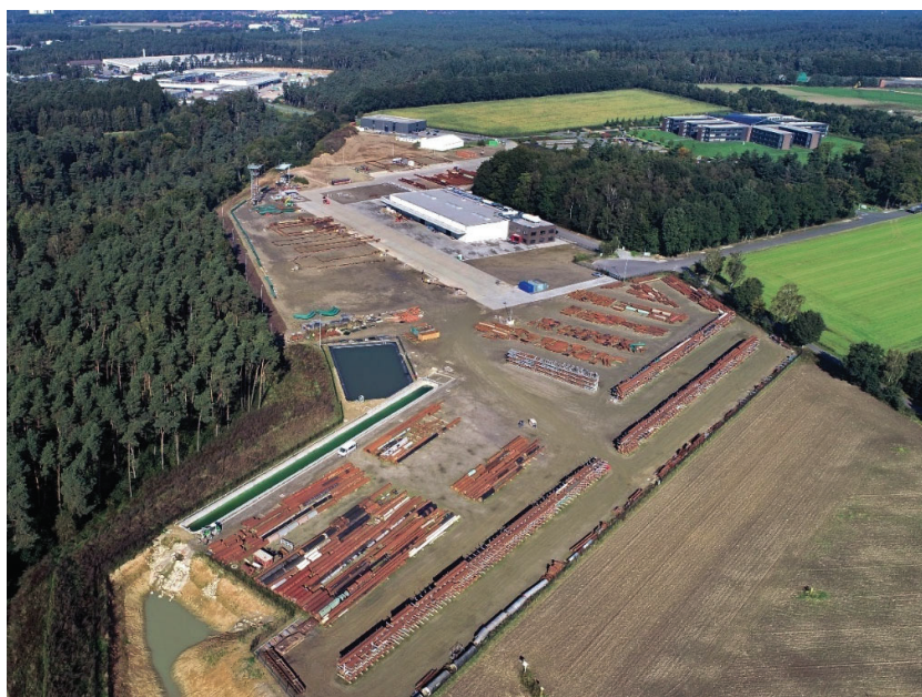
Figure 8. Aerial view of the ROSEN Test Centre in Lingen, Germany
