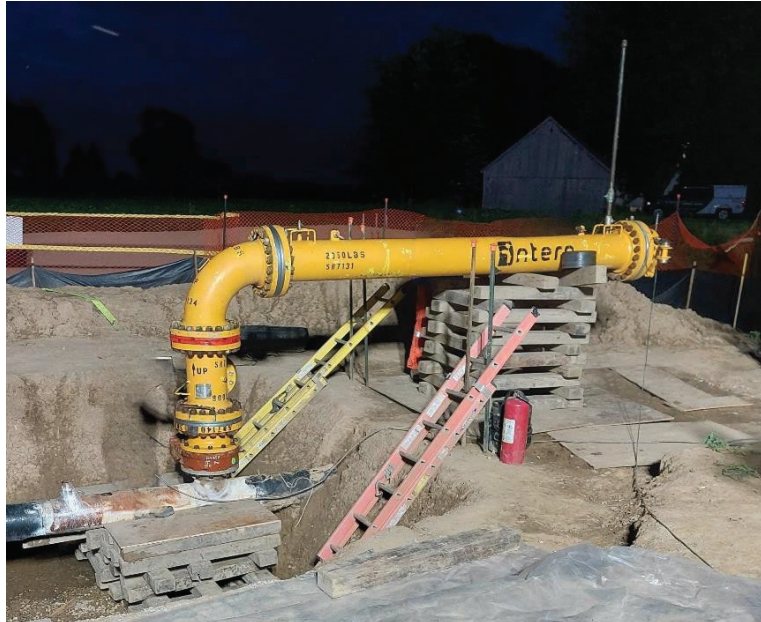
Figure 5. NPS 12 launch and receive site with Intero temporary launcher | Rural site
