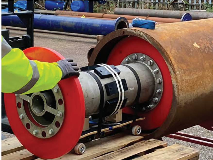
Figure 5. Test pig being inserted into the pipe
