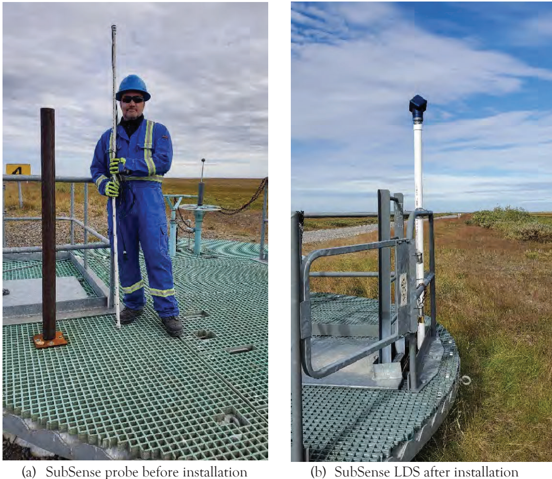
Fig. 8 Installation of SubSense LDS
