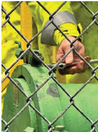
Figure 8. Gloves should be used when there is a potential for contaminants such as NORMs
