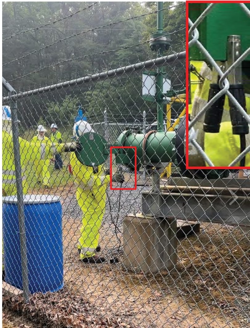
Figure 5. Never establish electrical connection while the trap door is open
