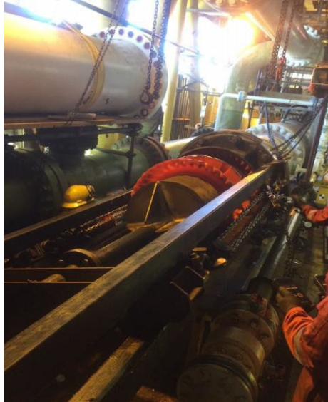
Figure 5: Rescue pig loading
