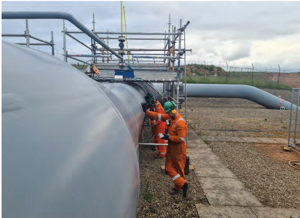
Figure 7. Close monitoring of tool location at receiver
