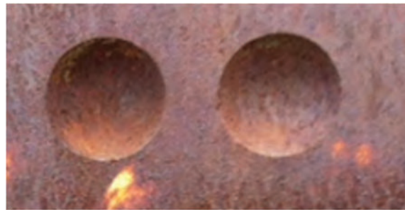
Figure 12a: Axially aligned pits
