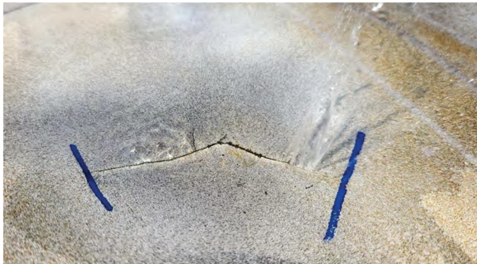
Figure 16. Close-up Photograph of the External Surface of the Pipe Section Containing the Case 4 Dent during the Hydrostatic Pressure Test Showing the Leak Location
