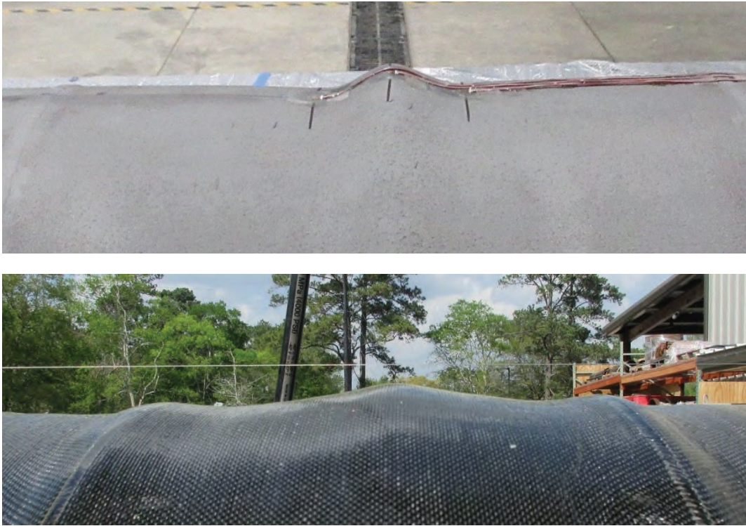
Figure 3. Wrinkle pre (top) and post (bottom) repair with carbon fiber
