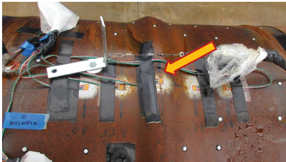
Figure 14. Photograph showing leak that developed in peak of the wrinkle bend
