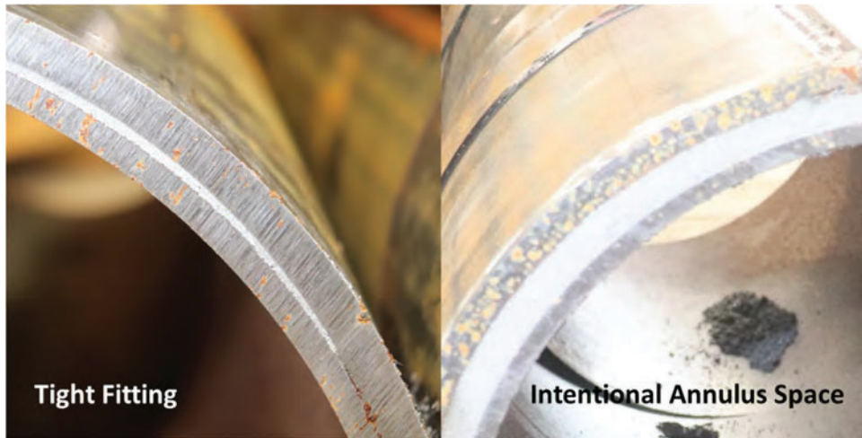
Figure 9. Resultant Five Star Fluid Grout 100 fill.
