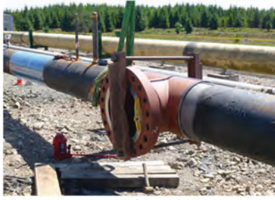
Figure 14. Setting up slit tee for welding at DNV Spadeadam
