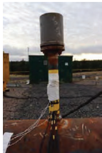
Figure 19. WP1 Tee Fatigue Test Vessel
