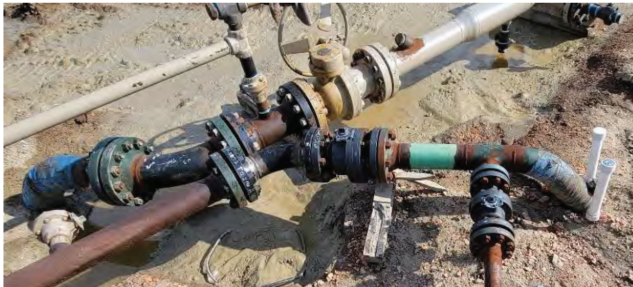
Figure 21. Closeup of 4" receiver and 6" launcher.
