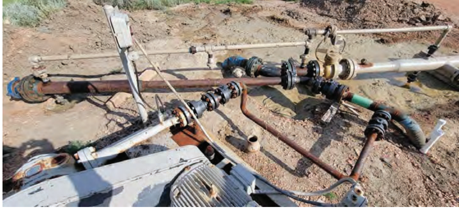
Figure 20. Installation of 4" receiver and 6" launcher at 4"/6" transition point of pipeline.
