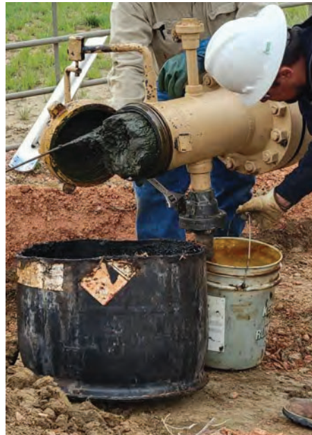
Figure 7. Paraffin wax “plug” in front of tool at receiver.
