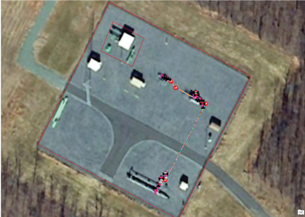
Figure 8: Aerial of Transmission Station in GIS Environment
