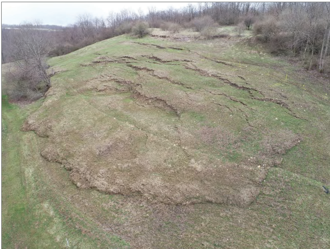
Figure 1. Example landslide crossing pipeline ROW, identified and remediated by Marathon Petroleum
