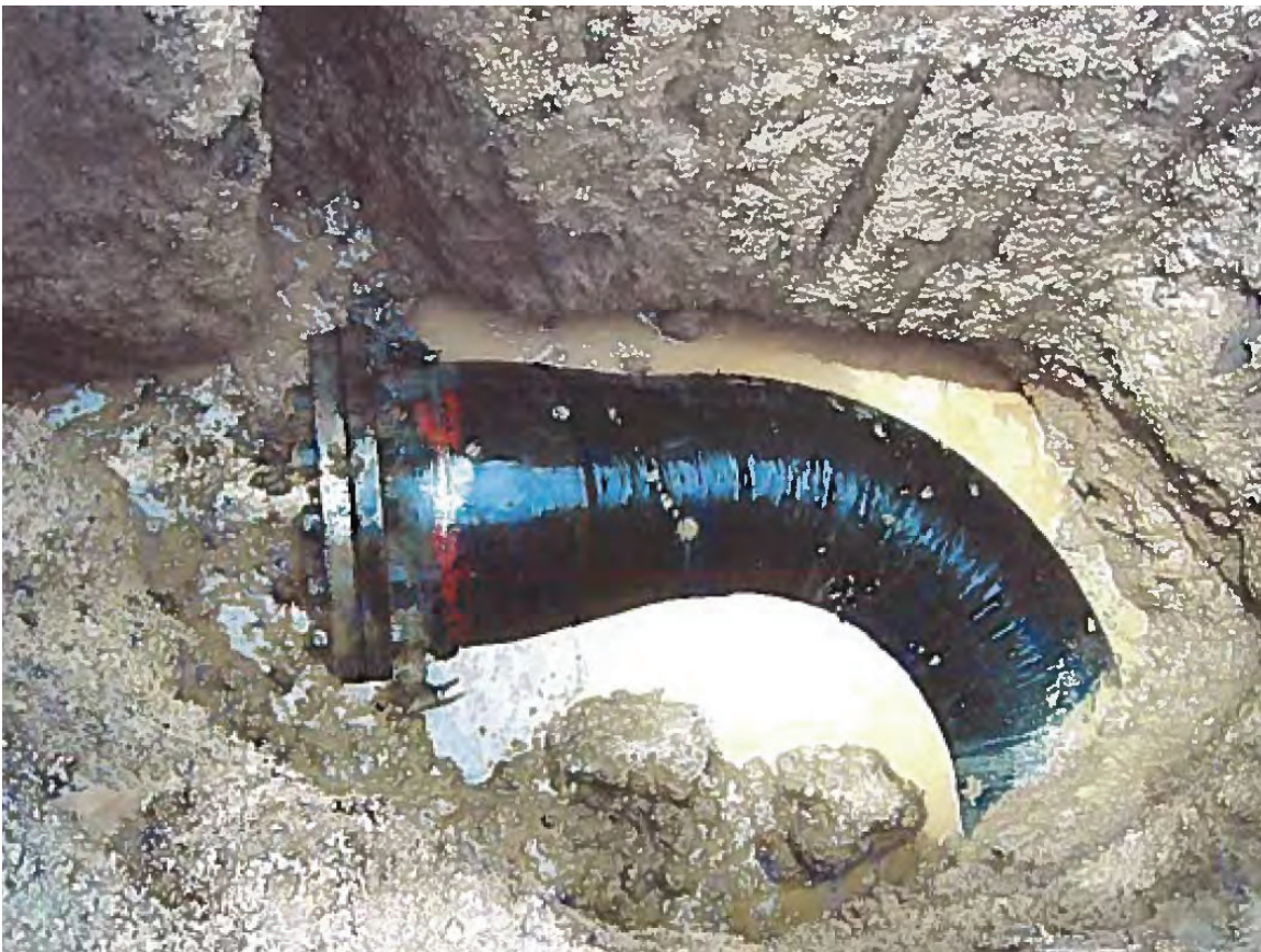
Figure 2. 16"/20" transition with affixed bend
