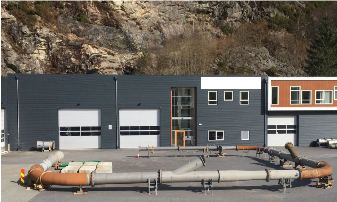
Figure 11. Pump trial setup including diameter change and Wye passage
