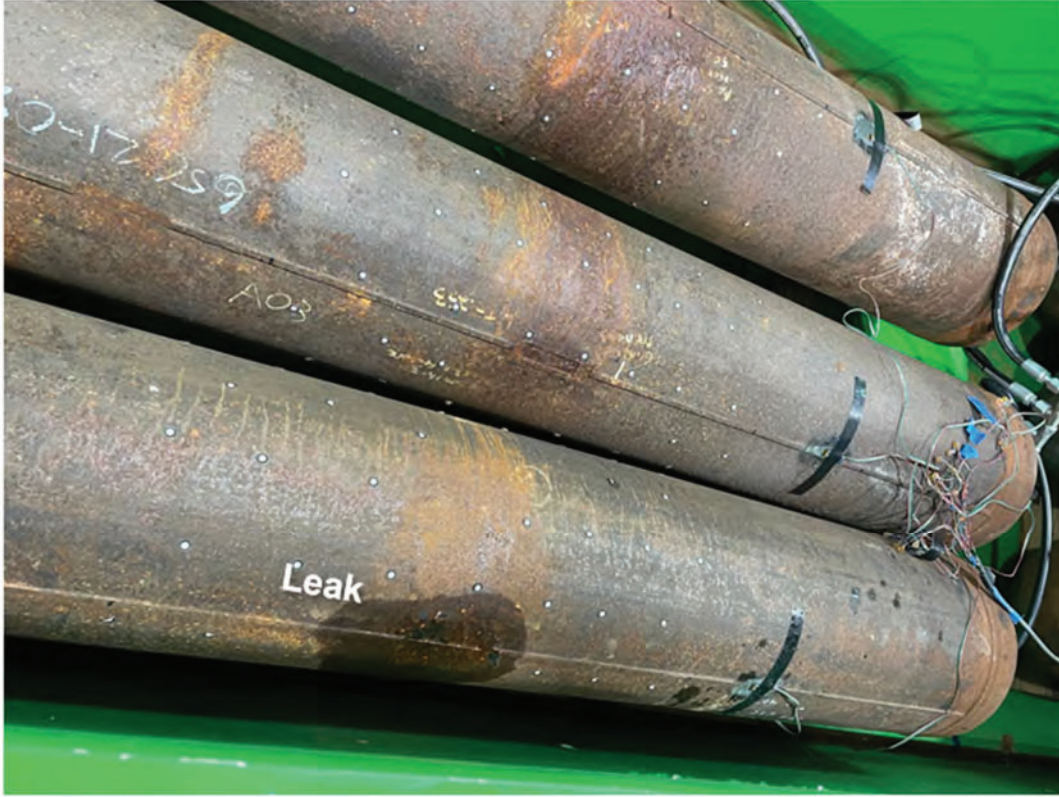
Figure 2. Leak observed in sample AO2 after 17,749 cycles.
