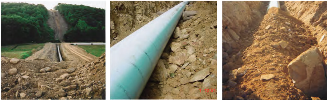
Figure 4. Images illustrating rocks in rights-of-way as potential sources of rock dents
