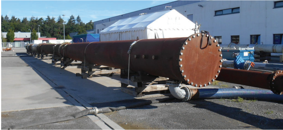
Figure 16. Pump test facility in Stutensee, Germany
