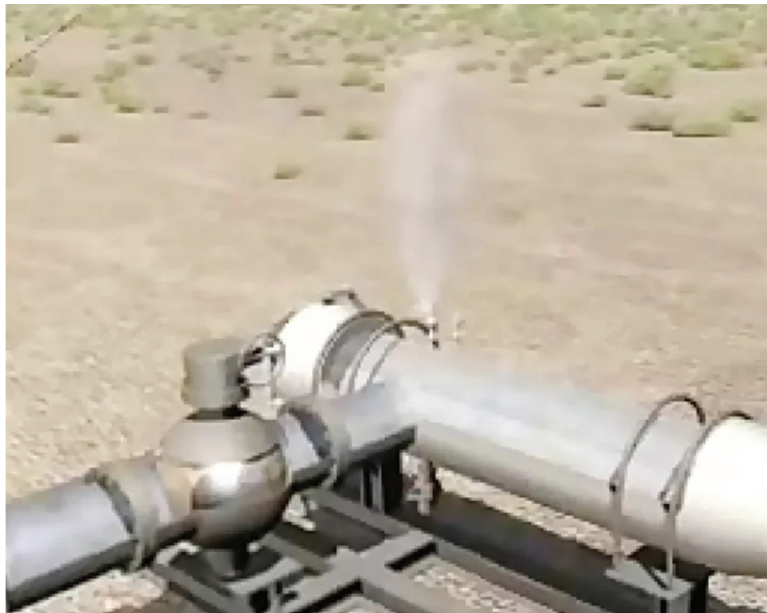
Figure 2. Debris from pipeline.
