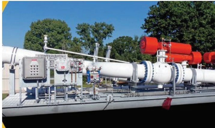
Figure 6. Pipeline trap components
