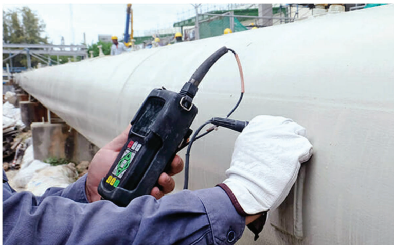
Figure 5. Measuring wall thickness.
