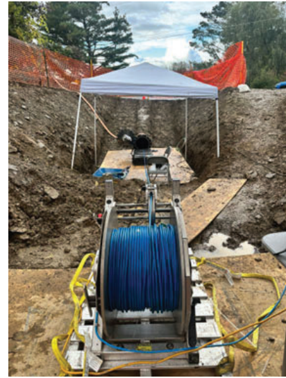
Figure 11 Onshore tethered pipeline inspection
