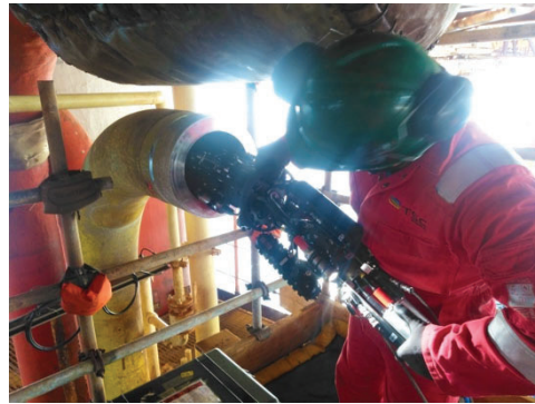
Figure 9 Offshore operation showing TRITON entering the riser.
