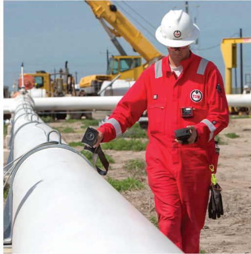
Figure 7: Pig tracking with handheld SmartTrack transceiver
