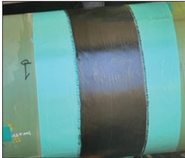
Figure 18. Nonmetallic composite repair in the field.
