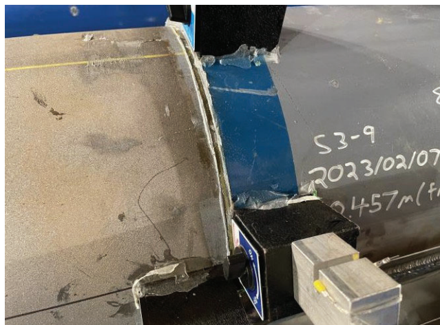
Figure 10. At the failure point where crack opened
