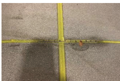
Figure 13. Illustrating Specimen 4-1A 80% Crack
