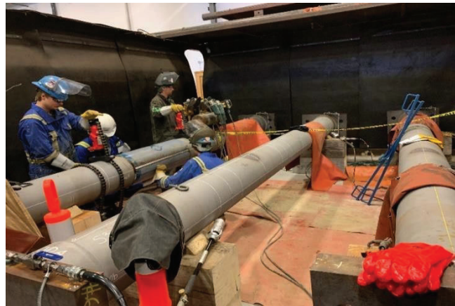
Figure 8. Installing Repair F
