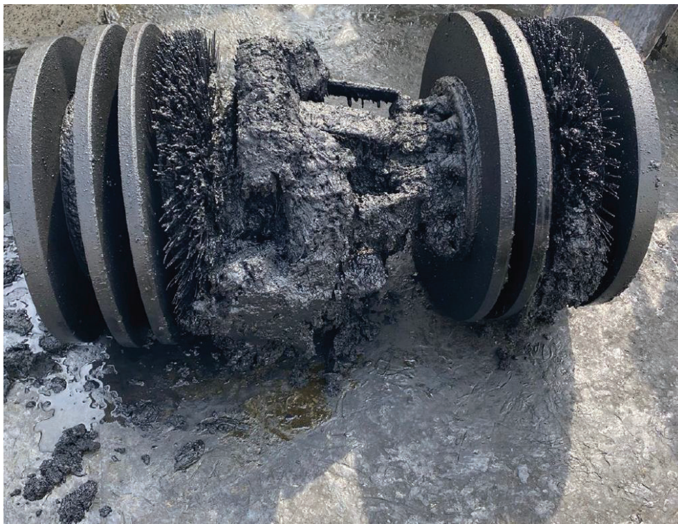
Figure 10. Last cleaning tool (After run)
