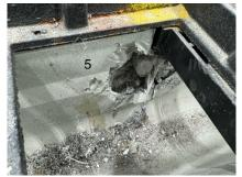
With Hole 5, the gap behind the hole was filled with urethane foam. After the hole is filled, it is not necessary for the foam to be smooth. In this environment, the patch by itself is capable of handling all the stress that could arise. The patch is the critical component of RPRS.
