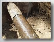
Sulfur hexafluoride (SF6) gas is injected into the hydrotest water throughout the filling process prior to
