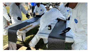
required to be "wetted out" before wrapping the repair. This procedure easily shortens smaller jobs by 30 minutes or more, while large-scale jobs could see time savings of up to several hours. As stated above, time saved is money saved when it comes to facilitating a quicker backfill.
