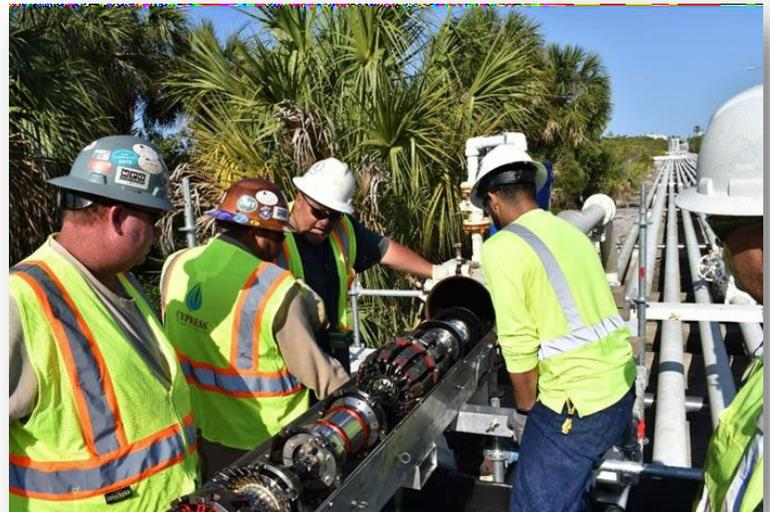
Tool being transported into launcher
