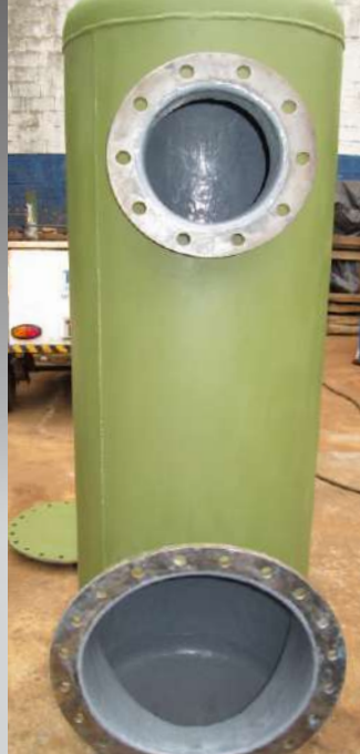
Repair and coating of pressure vessels
