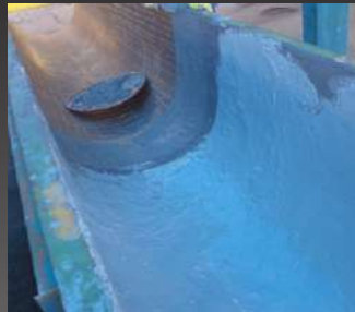
Coating of ditches
