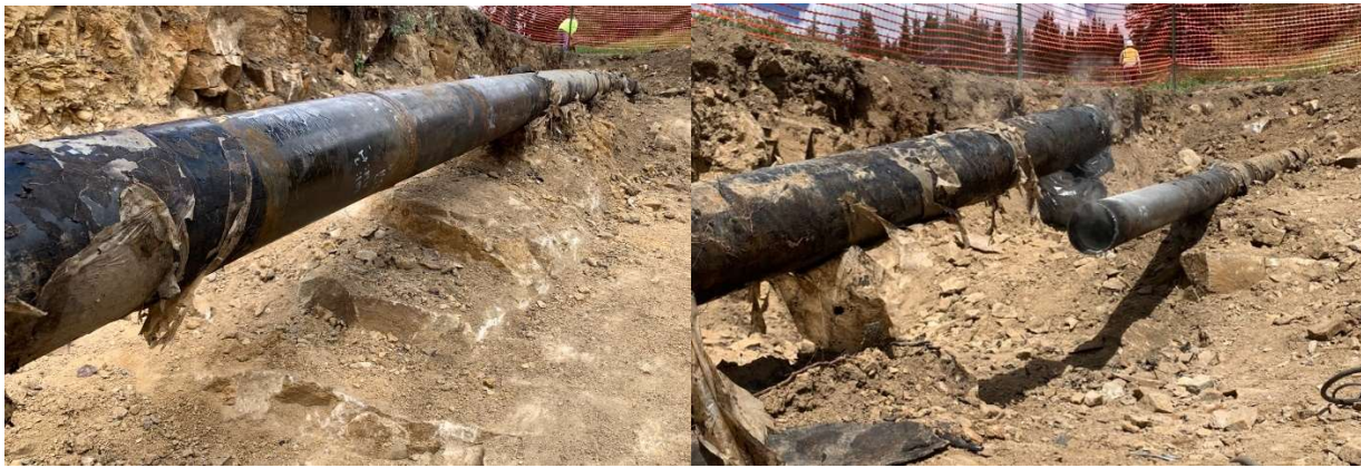
Figure Nine: CSCC Indication Excavation Before and After Initial Pipe Cut
