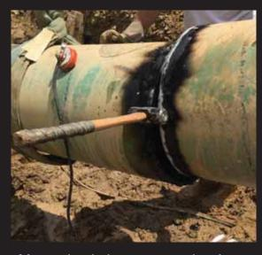
Magnetized pipes are a pain. Arc blow can cause weld defects and frustrated welders. Welding rod and metal tools can stick. These all add up to delays on your project.
