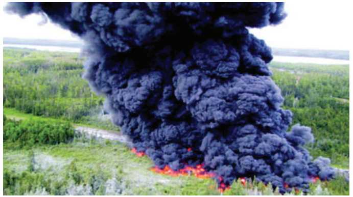
Figure 4. 34-inch diameter steel pipeline ruptured in Cohasset, Minnesota, on July 4, 2002.
