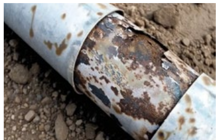
Figure 6: Excavation and verification of active corrosion using CMI
