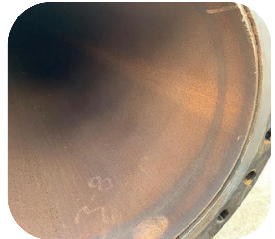
Pipeline, post brush cleaning
