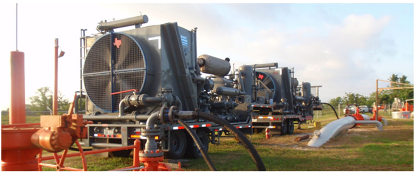
Compressors evacuating pipeline
