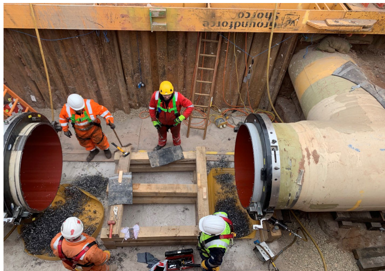
Clamshell Cutting Operation complete, 48" IJ Removed
