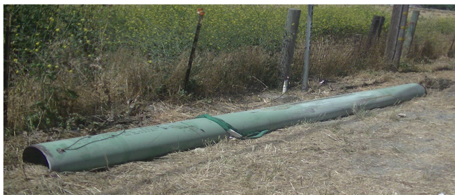
FIGURE 8. FBE-coated test pipe connected to ETS 451.54
