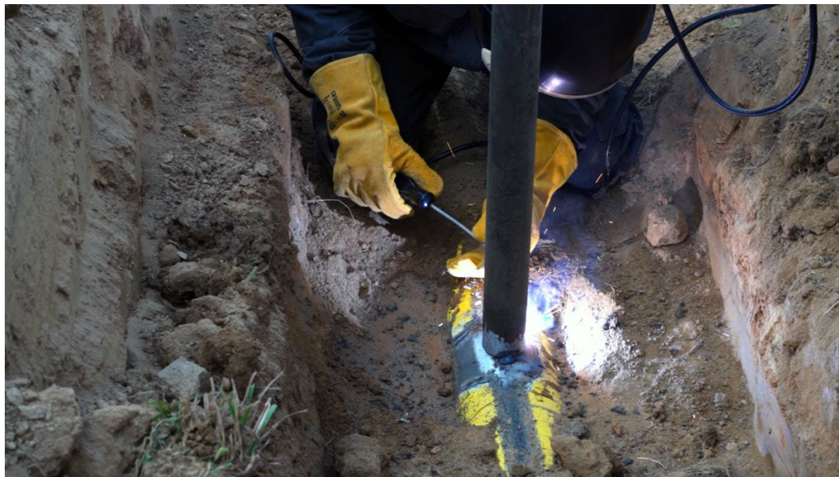
FIGURE 11. Tapping on the test pipe at Chameyrat
