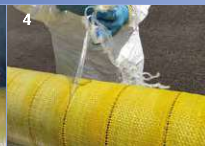
Remove compression film after full curing
