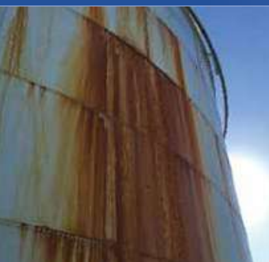
EXTERNAL CORROSION
