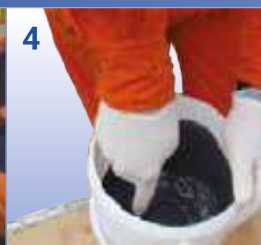
4 3X bi-component epoxy resin preparation
