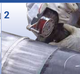
2 Surface preparation Sa2½ / St3 & roughness Rz > 60 µm (2.4 mil)
