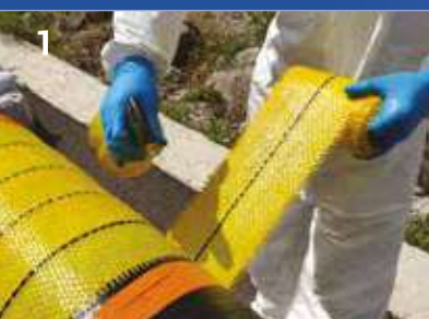
R1D wrapping (spray water continuously)
