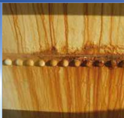
INTERNAL CORROSION
