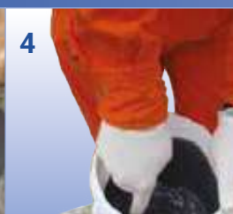
4 3X bi-component epoxy resin preparation
