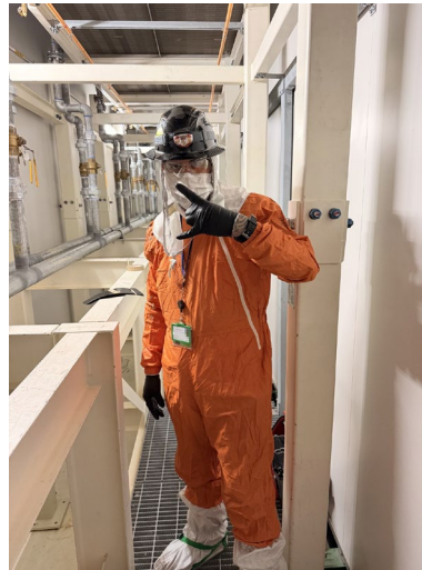
RT Technician @ Data Center
