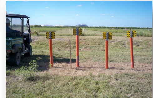
Pipeline Marker Placement
