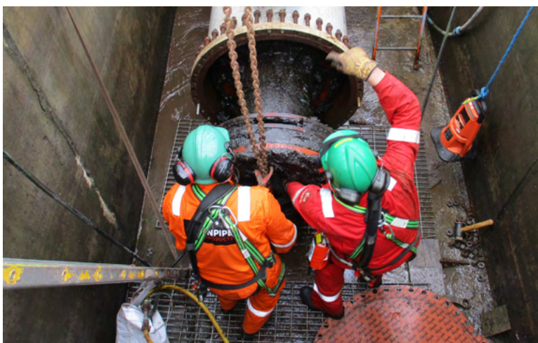
36" Pipeline Cleaning
