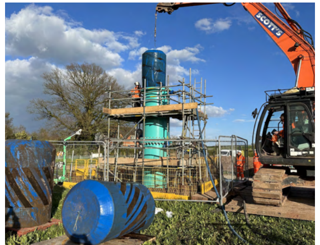
42" Water Mains Pipeline Cleaning
