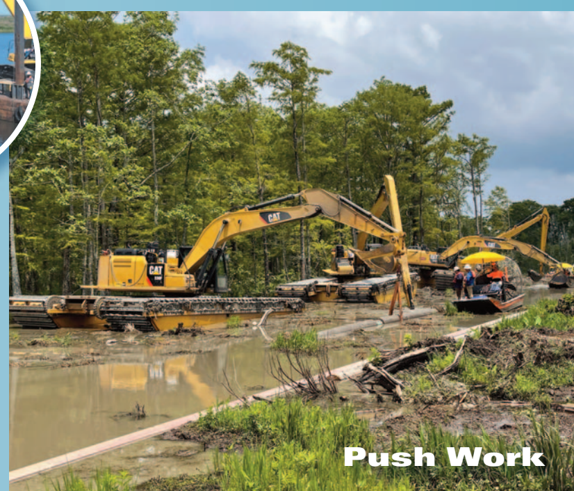
Sheet Pile Installation
